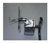
3. Thread the wires through the wall plate.
